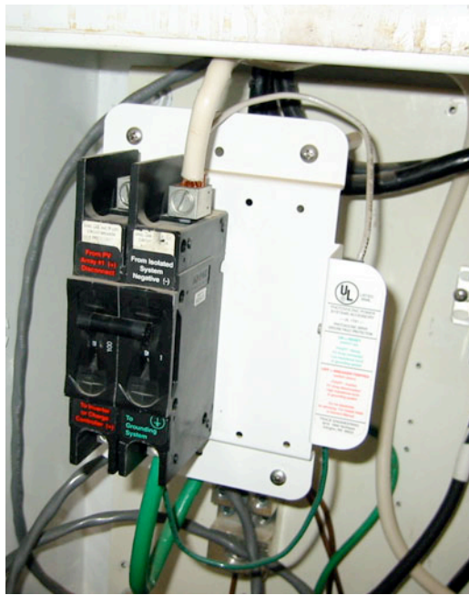
Figure 12. External Ground-Fault Protection Device
