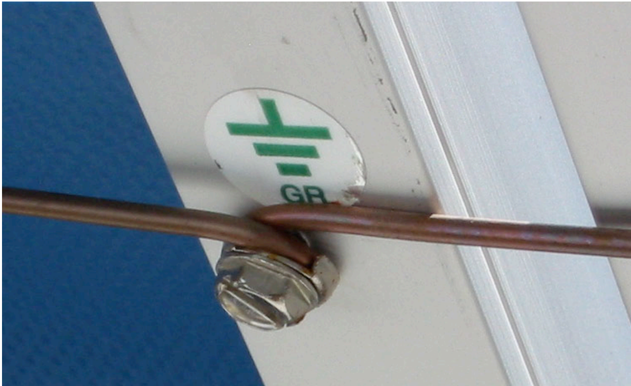
Figure G-3. Improper Module Grounding
